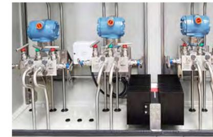
The cabinets and boxes can be fully prepared for any provided equipment, like analyzers for sampling conditioning systems.
