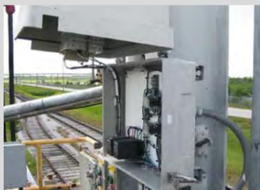
To create uniform conditions inside an enclosure, INTERTEC makes sure that they are properly thermally insulated, heated and/or cooled, just like a building. Thermal bridges are particularly harmful, as temperature gradients and condensation in these areas endanger the function of installed electronics.
